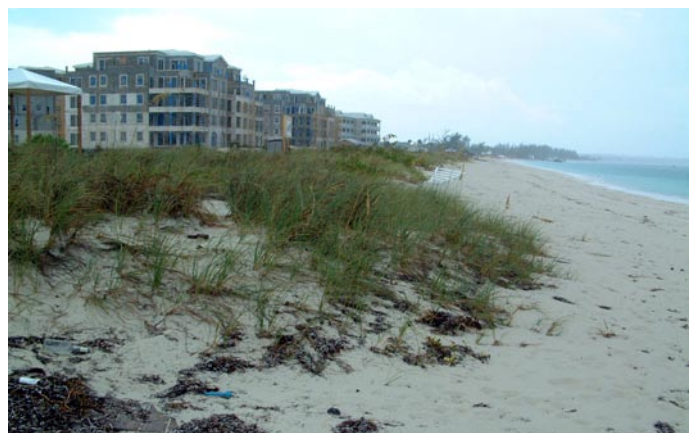
Photo 9.8. Development immediately adjacent to a beach within Princess Alexandra National Park, Providenciales (Photo P. Richardson).
